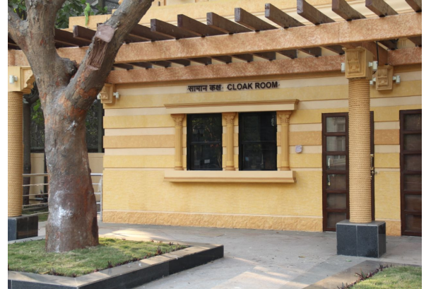
Public Toilet Facility
